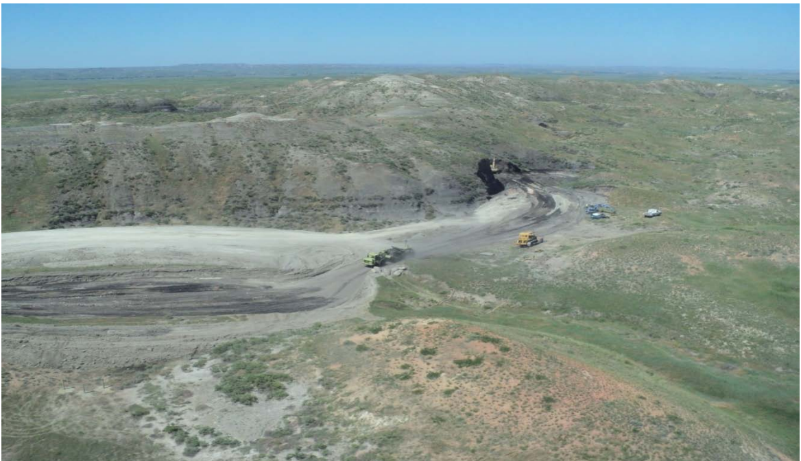
Figure 10. Aerial view of the Tonn #1 Outcrop Fire showing outcrop excavation and repository area for mixing embers with overburden prior to burial.
