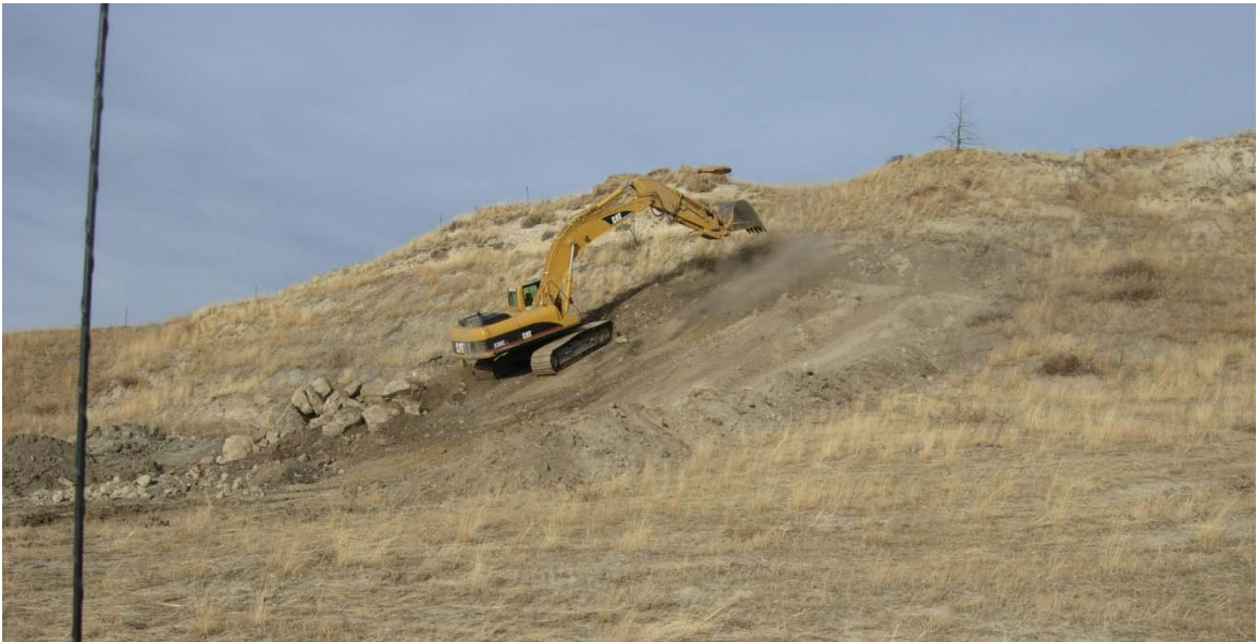
Figure 5. Charter Coal Mine Fire in early excavation phase.
