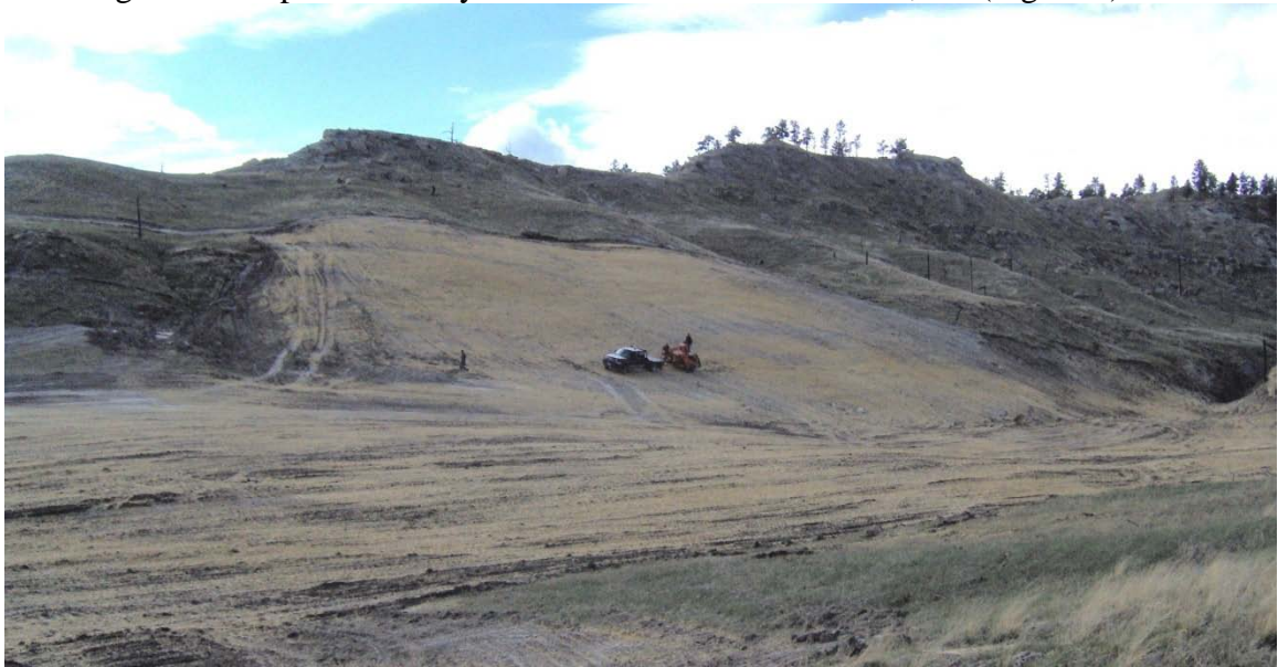
Figure 6. Marsh Outcrop Fire at final contour and mulching.
