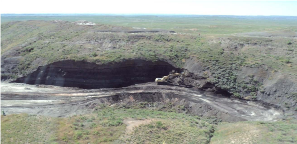
Figure 9. Aerial view of the Tonn #1 Coal Outcrop Fire with excavation exposing the burning coal bed at the face of the outcrop.
